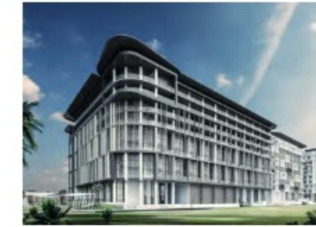
OASIS RESIDENCE TWO, MASDAR CITY
